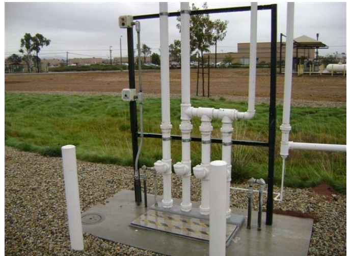
Tank Overfill Alarm next to UST Vents
