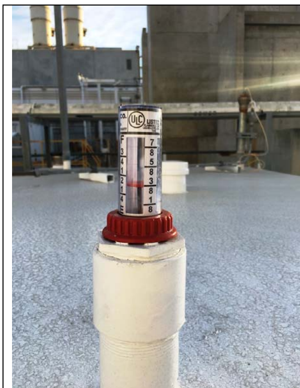
Mechanical Post Gauge
