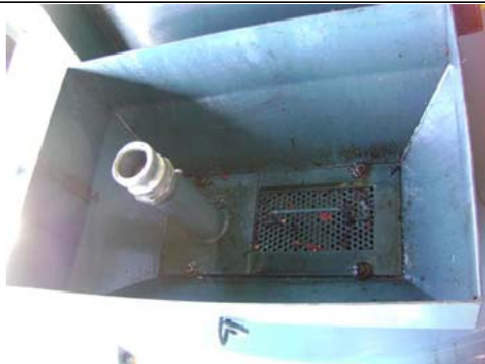
Round Covered Spill Bucket
