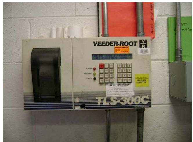
Veeder Root TLS-300C Alarm Panel inside Building 8545
