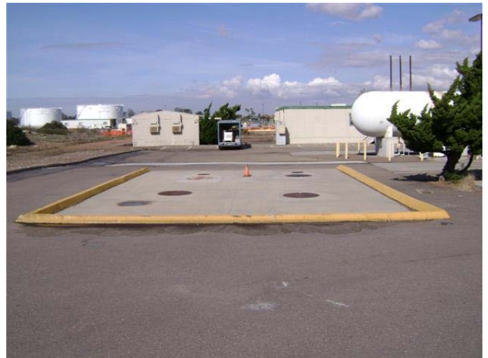
Location of USTs within Concrete Bermed Area
