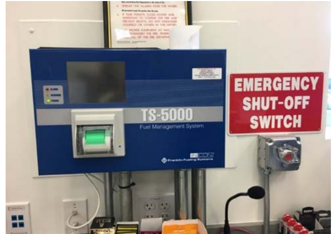
ICON TS-5000 alarm panel and emergency shut-off switch inside Building 8676
