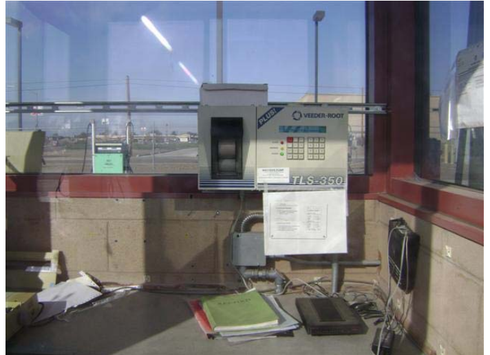
Veeder Root TLS-350 Alarm Panel inside Kiosk
