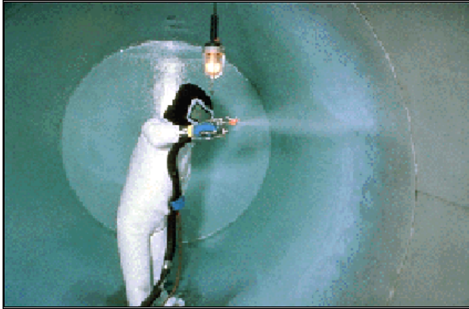
Figure 21: Application of an Internal Lining Within a UST
