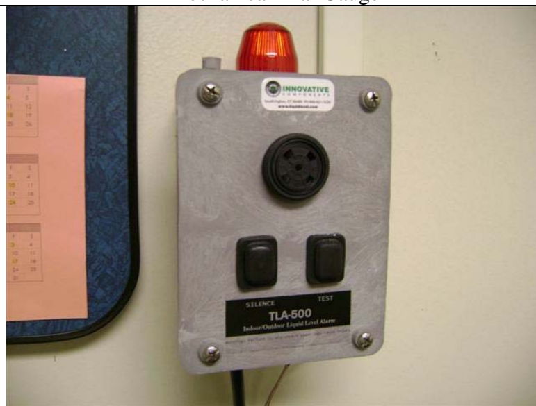
Electronic Level Sensor Alarm Panel
