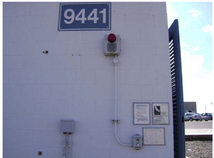
Exterior Building Alarm Light
