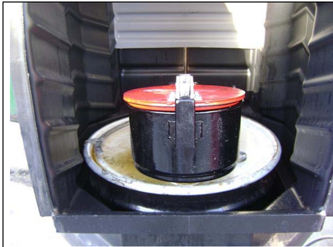
Round Covered Spill Bucket
