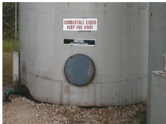
Category 3 AST – Single-Wall Tank with no Overfill Protection
