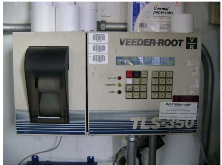
Veeder Root TLS-350 Alarm Panel inside Kiosk
