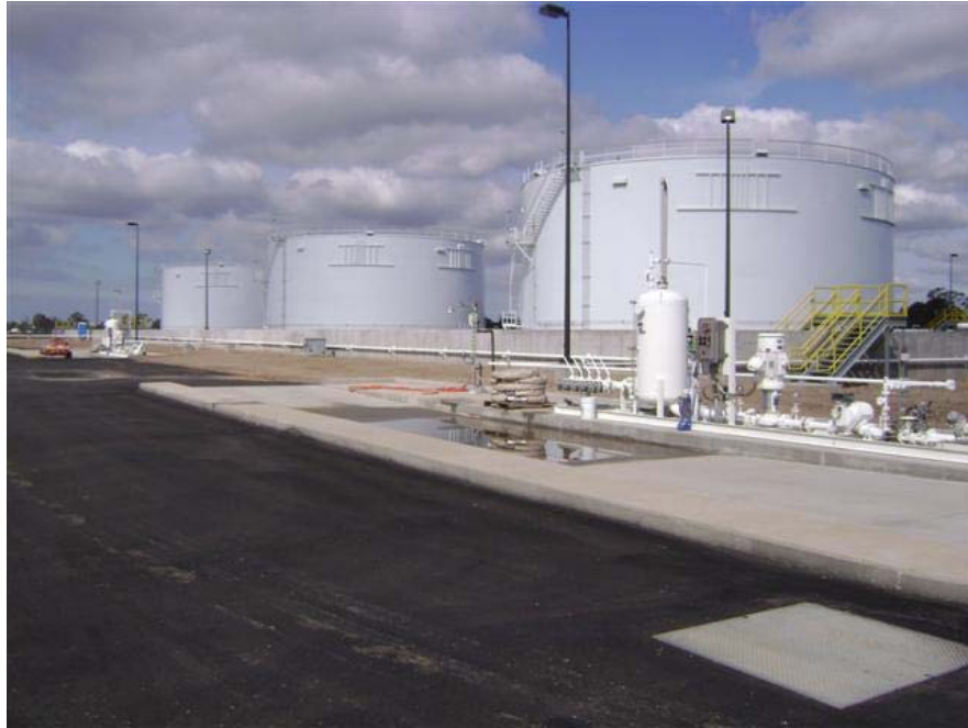
Figure 31: Example of Field Erected ASTs
