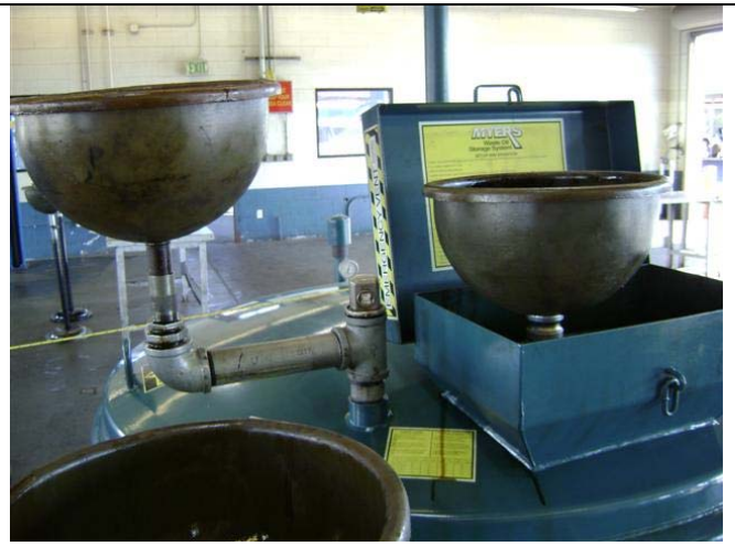
Secondary Round Spill Bucket
