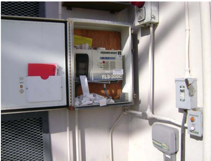
Veeder Root TLS-300C Alarm Panel
