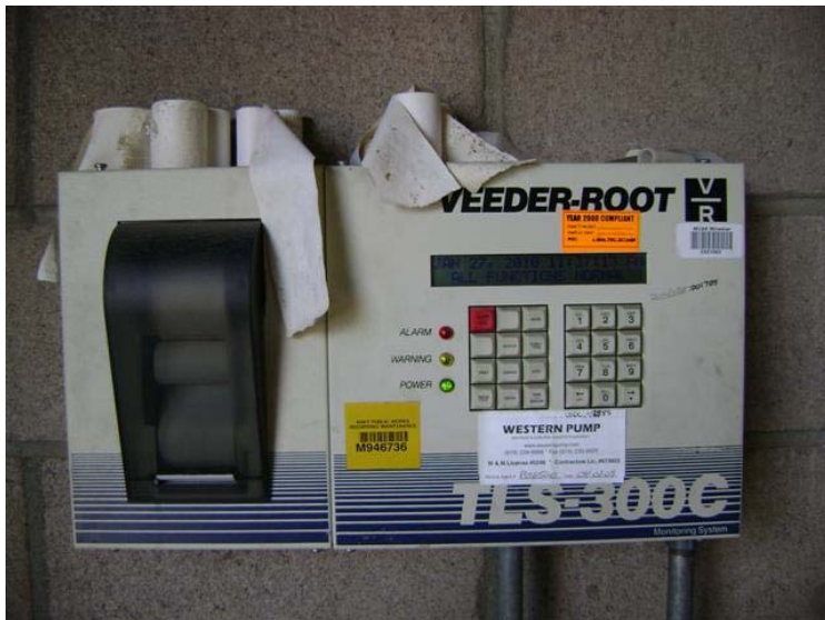
Veeder Root TLS-300C Alarm Panel inside Building
