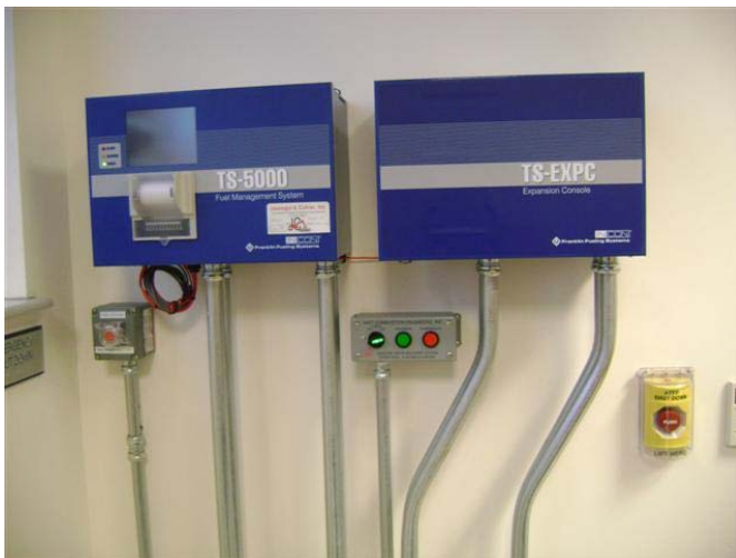
Incon TS-5000 Alarm Panels inside Building
