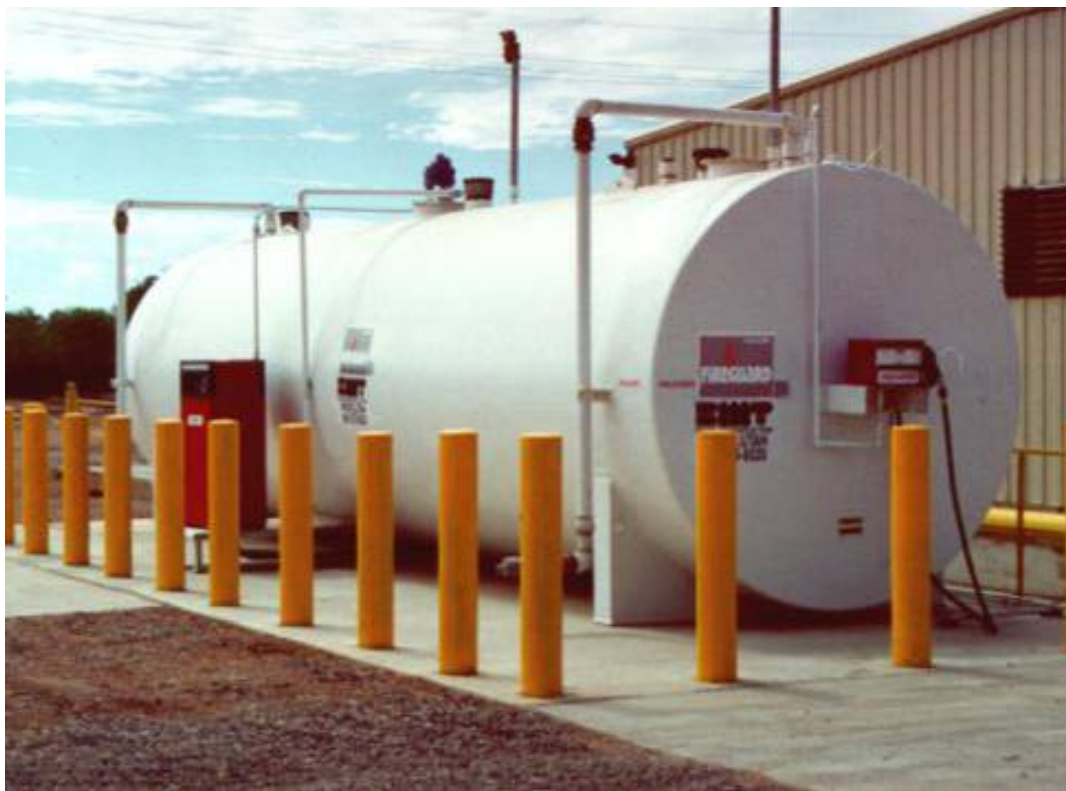
Figure 24: Example of Shop-Built AST
