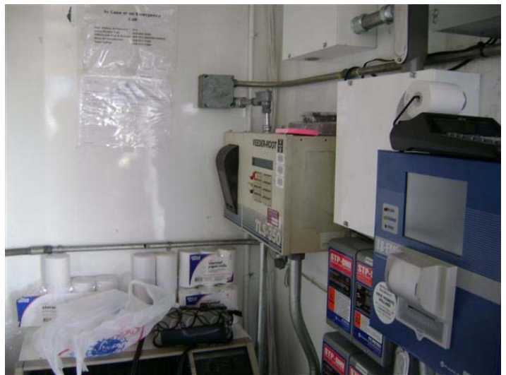
Veeder Root TLS-350 Alarm Panel inside Kiosk
