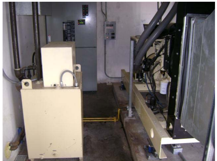
Interior Mechanical Room containing Day Tank and Emergency Generator
