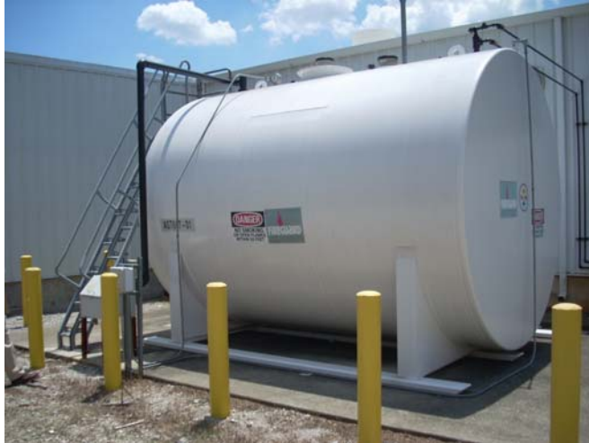
Category 1 AST – Double-Walled Tank with Overfill Protection
