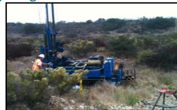
Drilling operations at IR Site 2
